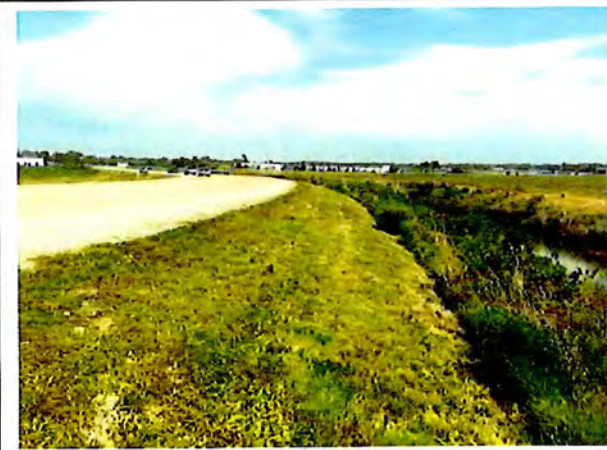
Steep shoulders and creek at a horizontal curve after a bridge
