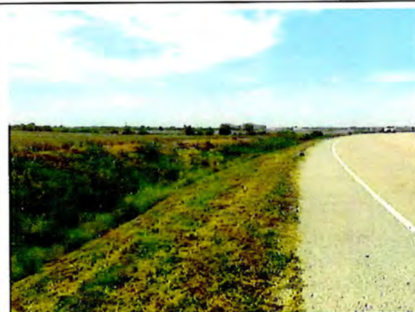
Steep shoulders and creek at a horizontal curve before a bridge.
